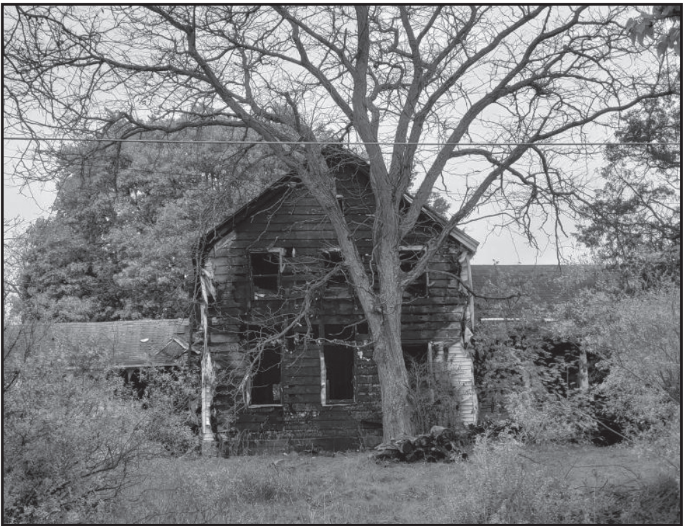
The fire that claimed one life and left another critically injured, took place at this house on Flat River Drive, a large, old, balloon-frame farmhouse, built before it became a standard practice to install flame-retardant material, or fire breaks, into the walls to help contain a fire.
