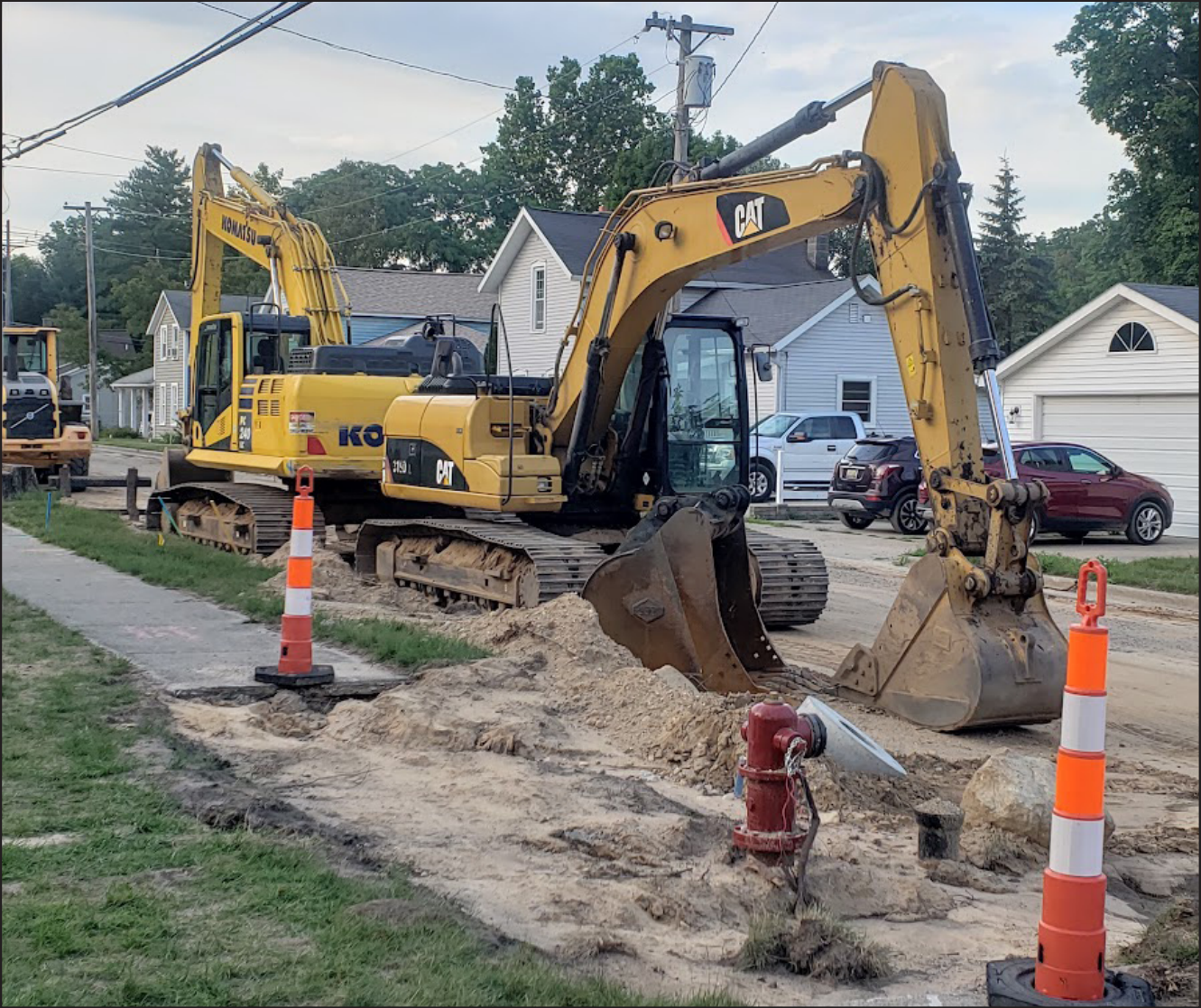
Roads, continued page 2 Big equipment for a big project.
