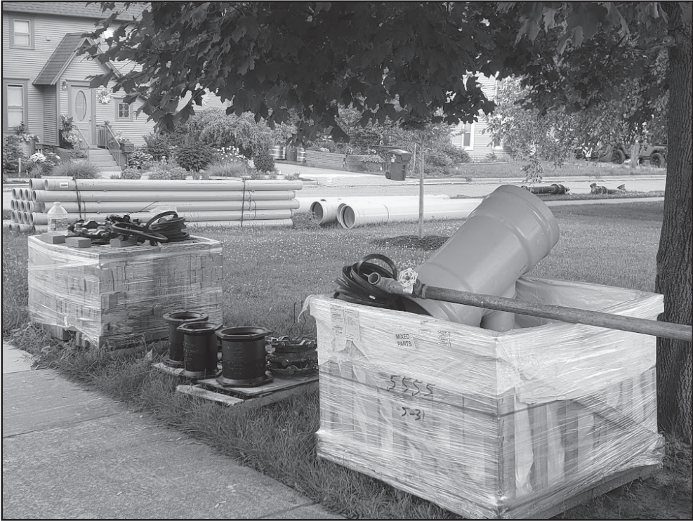
New water and sewer pipes are staged along Monroe Street.
