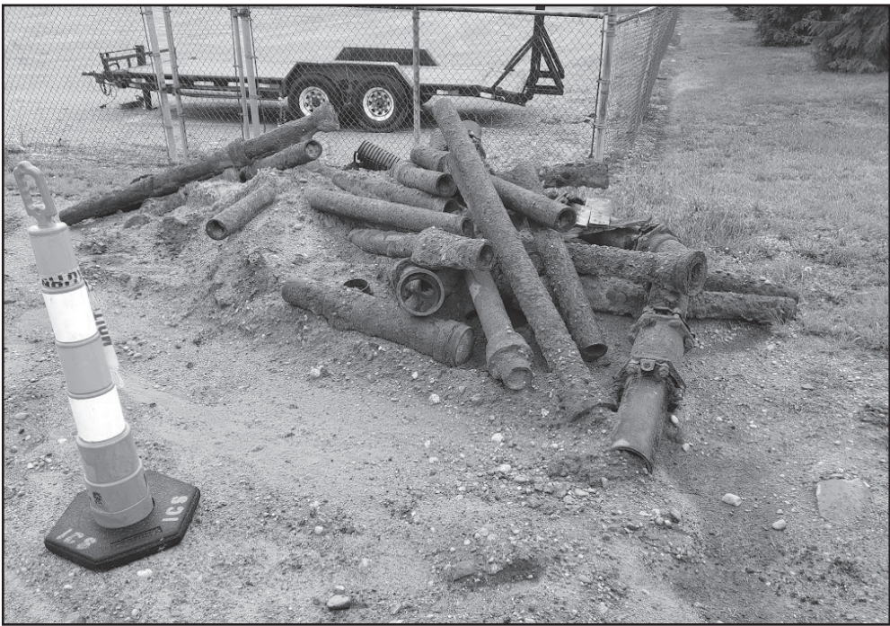
A sample of the water delivery system that is being replaced.
