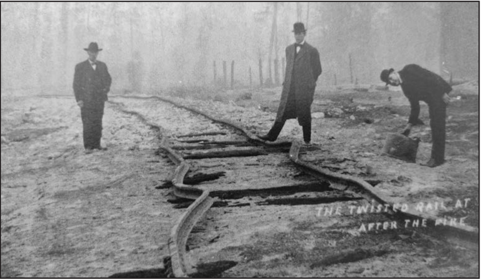
The warped tracks caused the train to derail. Sadly, most of the passengers perished. Photo Credit: Presque Isle Historical Museum
