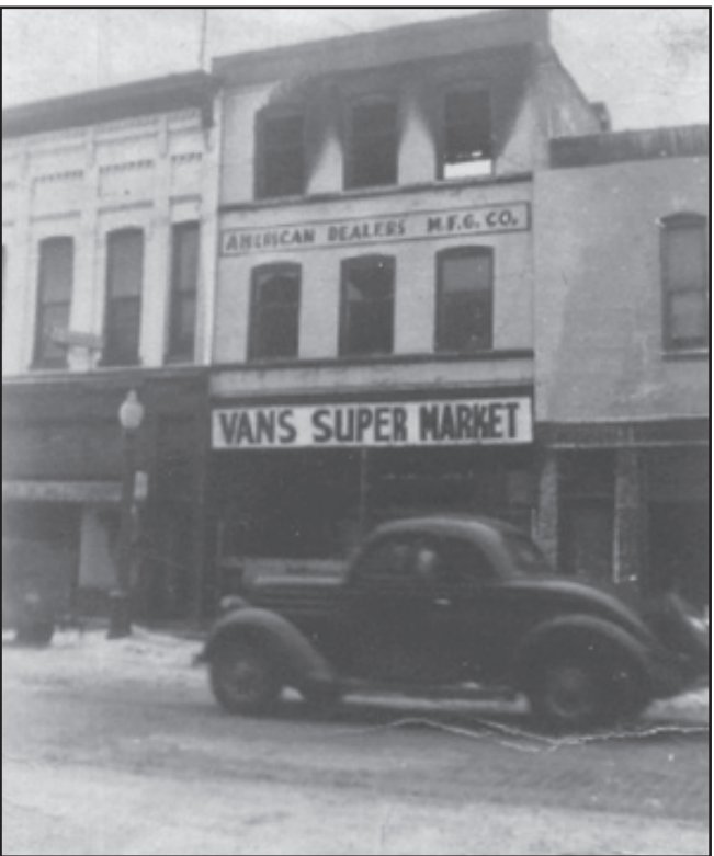
Photo taken after the fire of 1945 destroyed the 3rd floor. Van's Super Market had moved out and Al Hermans was trying to prepare for a Gambles store. The front reads "American Dealers M.F.G. Co."
