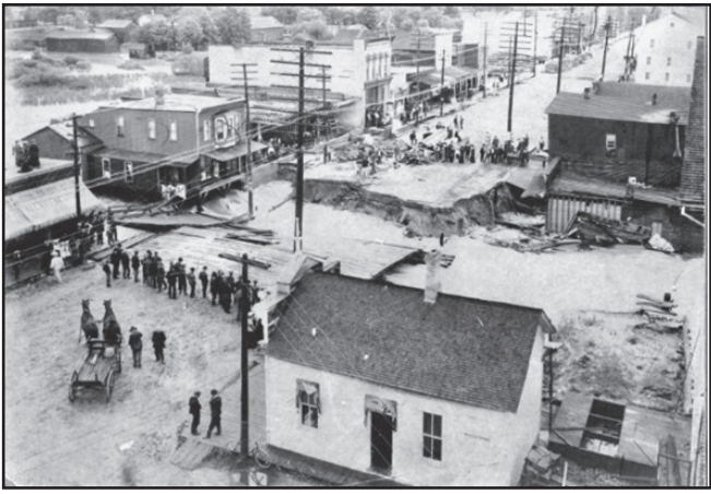
Main Street bridge was washed away in the Great Flood of 1905.
