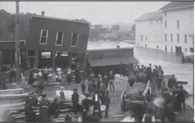
“Flood of 1905” photo shows 104 W. Main (the 2-story building) leaning.
