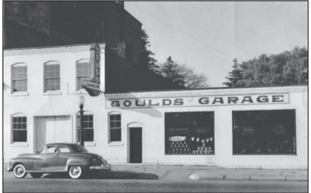
The one-story building on the right is 319 E. Main. Gould's Garage used both 317 and 319 East Main from 1925 to 1944; Peter Speerstra bought the buildings and kept the "Gould's Garage" name until he moved out in 1954.
