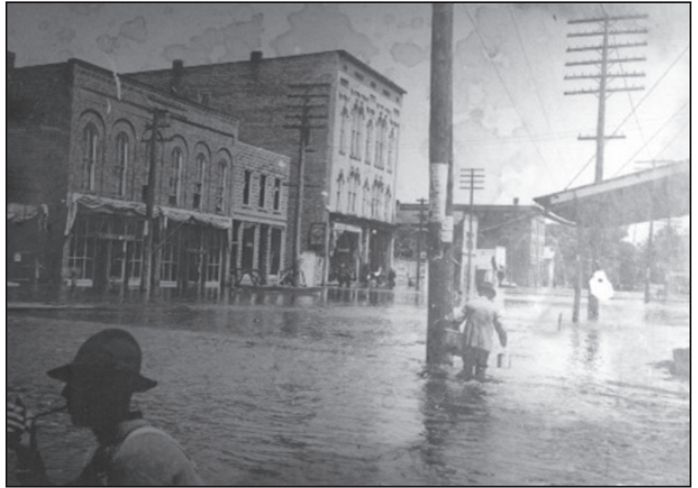
The cement block building was being built during the flood of 1905. The plate glass windows have not yet been installed. Notice the stylized cement blocks, which were popular during the early 1900s. You could purchase block-making machines from Sears and Roebuck Co.
