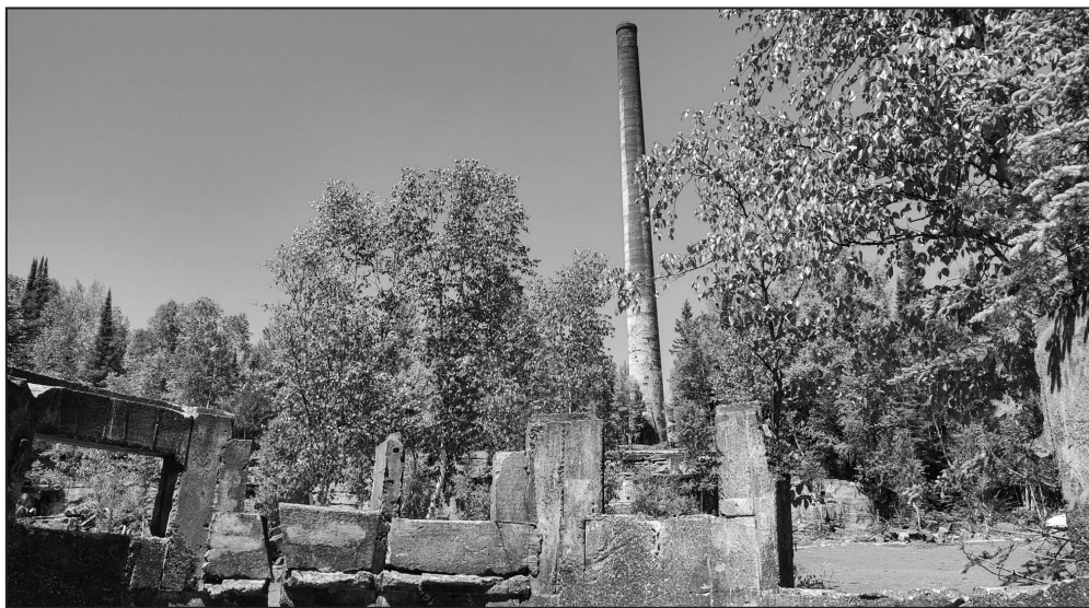
Built in 1901, the mill has been crumbling since its closure in 1932. The lone smoke stack stood quietly among the trees which had overtaken the stamping mill.
