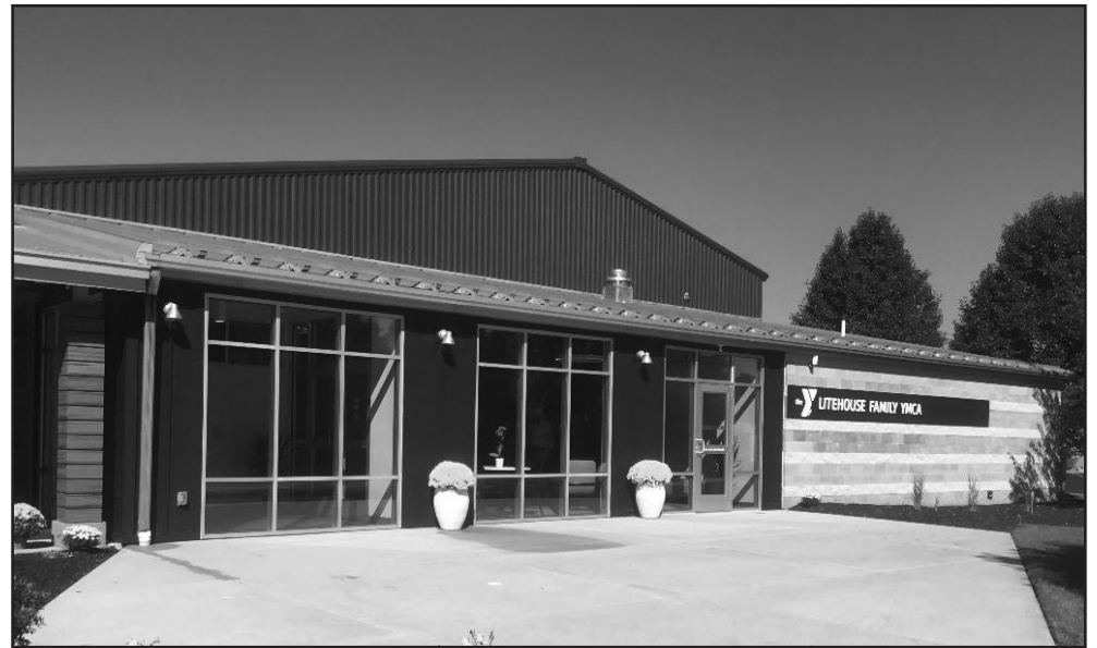
The new exteriors of the YMCA facility.
