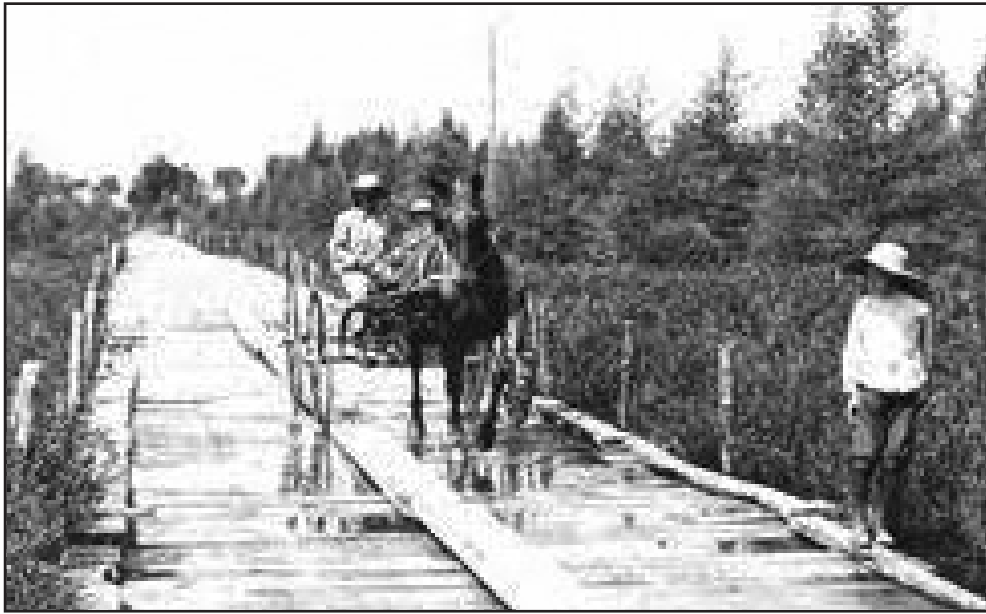
This is a plank road in Michigan. Photo Credit: History Grand Rapids.
