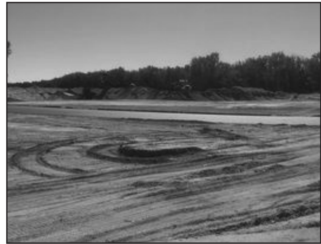
The mining on the south side of Bowes Road has begun.
