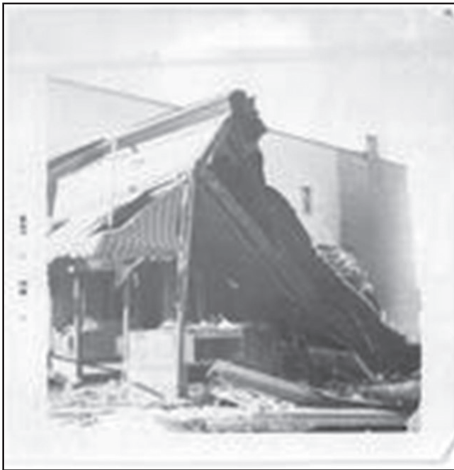
The remains of Molly Wepman's building after the fire of 1958. Molly and friends pulled smoke damaged goods out, cleaned them up and held a "fire sale". She paid her suppliers off, a little at a time, until every debt was settled.
