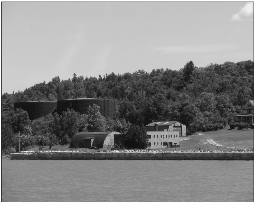
The two insulated fuel oil tanks held precious "Number 6" fuel.
