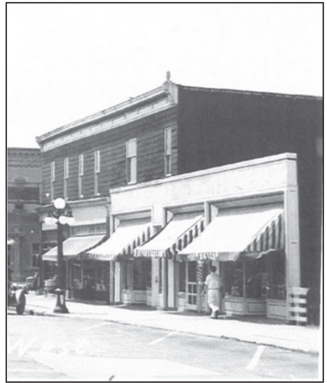
The three storefronts 115, 117, and 119 W. Main, notice the barber pole on the center storefront. Among the barbers were Jud Tinkler, John Bannan, Mabel Scott and Owen Ellis, Dick and Owen's, Stiles Beauty Shop.
