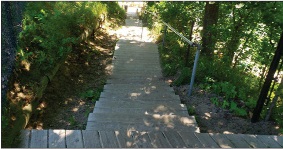
Top of the stairs looking down.
