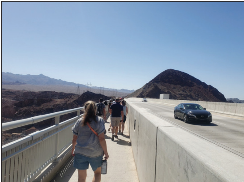
This is the walkway across the bridge.
