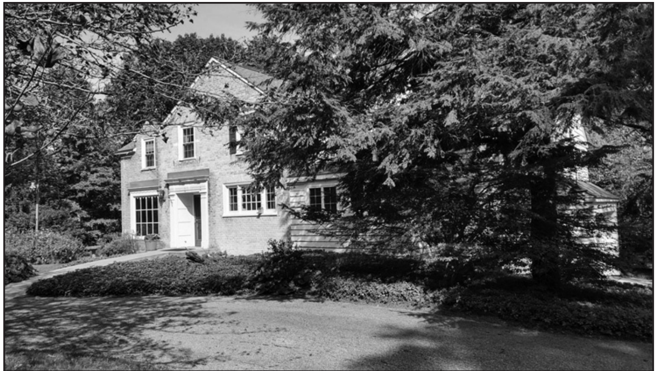
This estate home was built from 1936-1938. The Morton family invested in this land and helped to plant over seventy unusual trees on their property.
