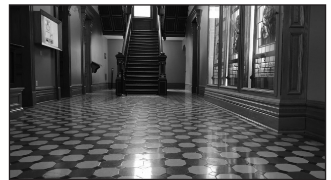
The entrance to the prison. The tiles are original. The Portuguese manufacturer is still in business and will provide new tiles if needed.
