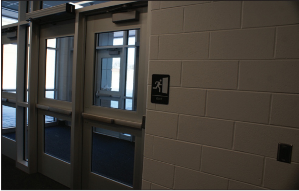
Next year, this will be the door where visitors enter.
