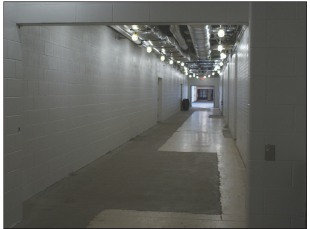
Some areas are still under construction.
