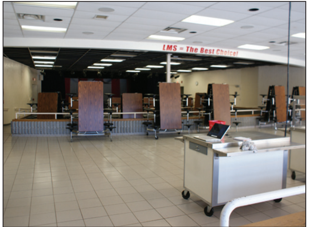
This will be the site of a new auditorium.
