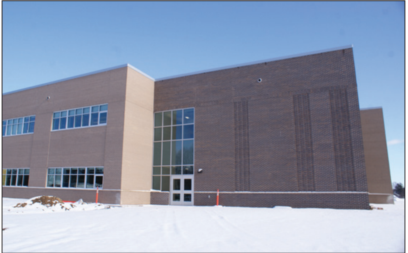
Exterior view of the new two story addition to Lowell Middle School.
