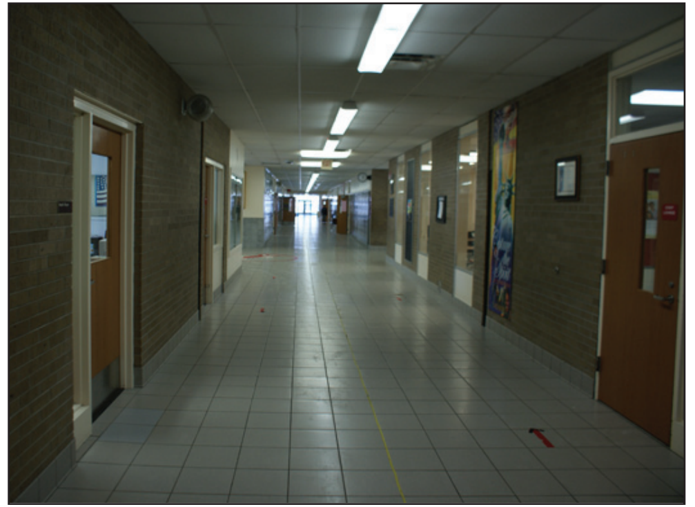
This old hallway will be demolished.
