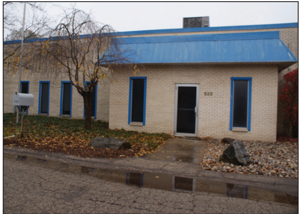
533 Godfrey the day after the fire.
