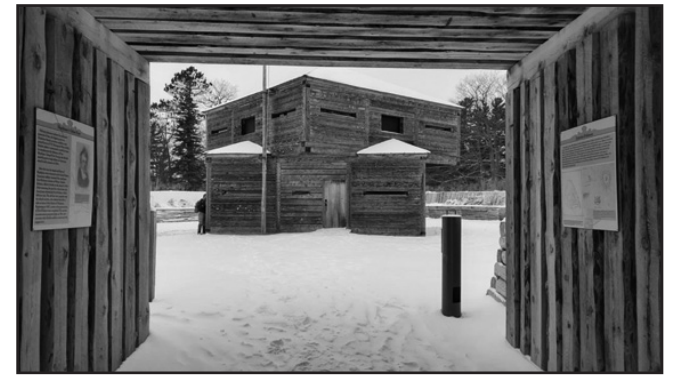
In 1814 Fort George was built by the British at the highest point on Mackinac Island, honoring King George III. The inner structure allowed for a wide-scope view of the straits. Funds to rebuild this structure for its bicentennial were appropriated in 2014.
