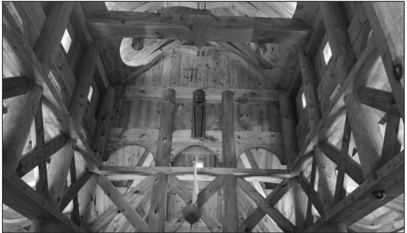
The hand hewn logs with tongue and groove joints support the structure. The 13 windows at the top allowed for natural light. Otherwise the only other light source would have been candles and lanterns.
