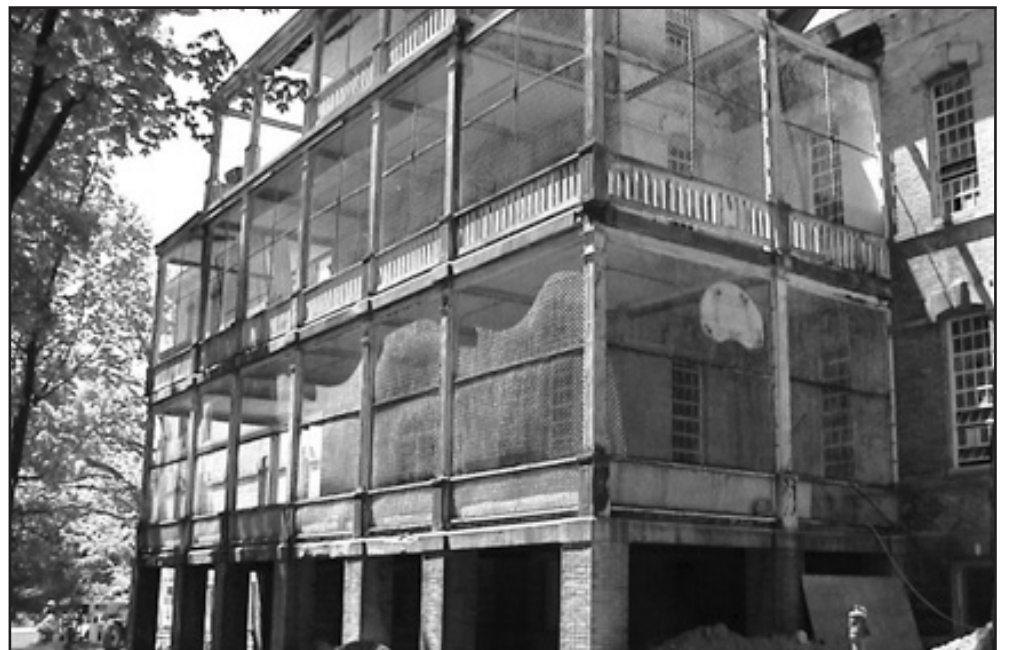
This is a 'screened porch' at the Traverse City State Hospital. The 'screen' is actually welded metal forming a cage-like enclosure.
