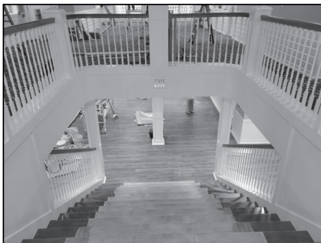
Freshly painted interior stairs. [photo by Wolverine Building Group]
