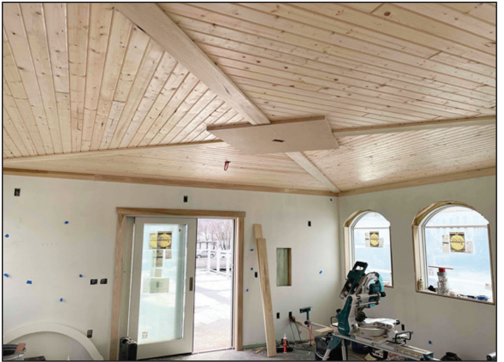
Brand new "tongue and groove" ceilings in the wheelhouse.
