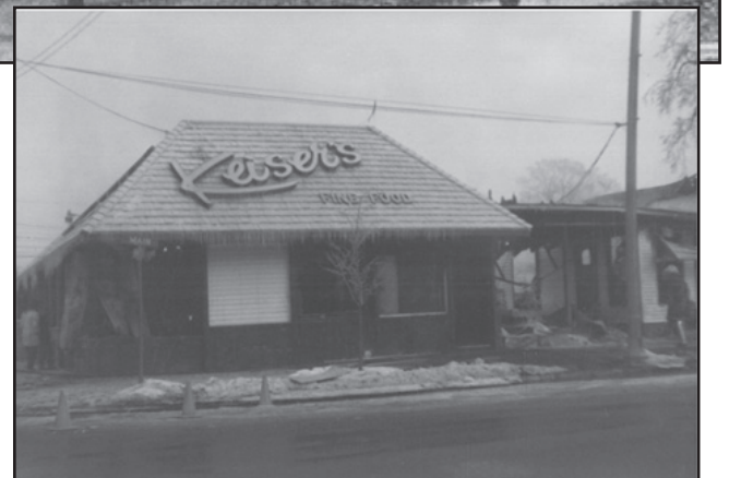
Keisers in 1988 after the fire.
