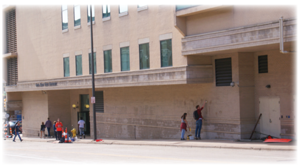
Volunteers and business owners spent most of the weekend washing off the graffiti and boarding up all of the broken windows downtown. This photo was taken on Saturday afternoon.
