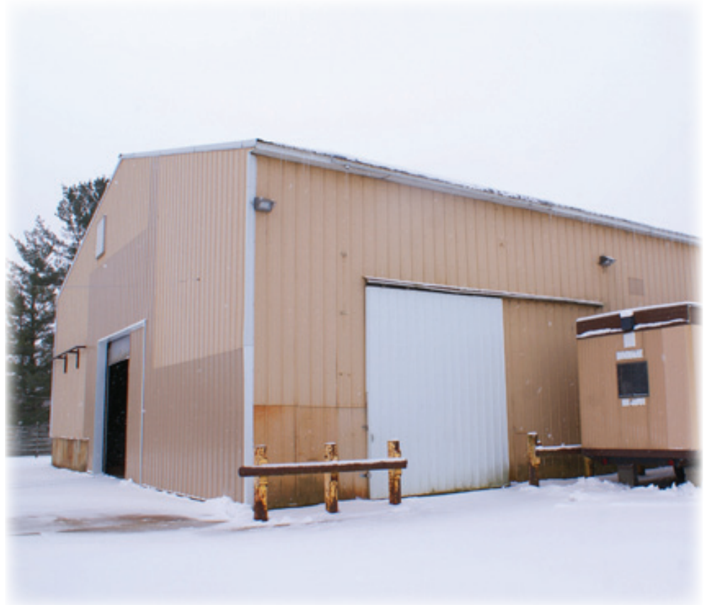
The Red Creek Waste Services facility on Main St. is not equipped to handle drop-offs of household recyclable items.
