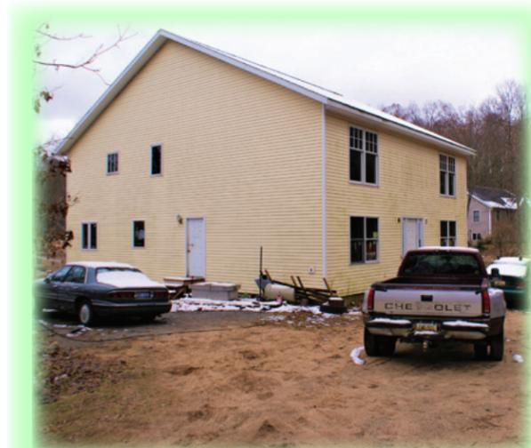
This home on Foreman is almost finished, it just needs some drywall, a basement floor, the furnace installed and some light plumbing work.
