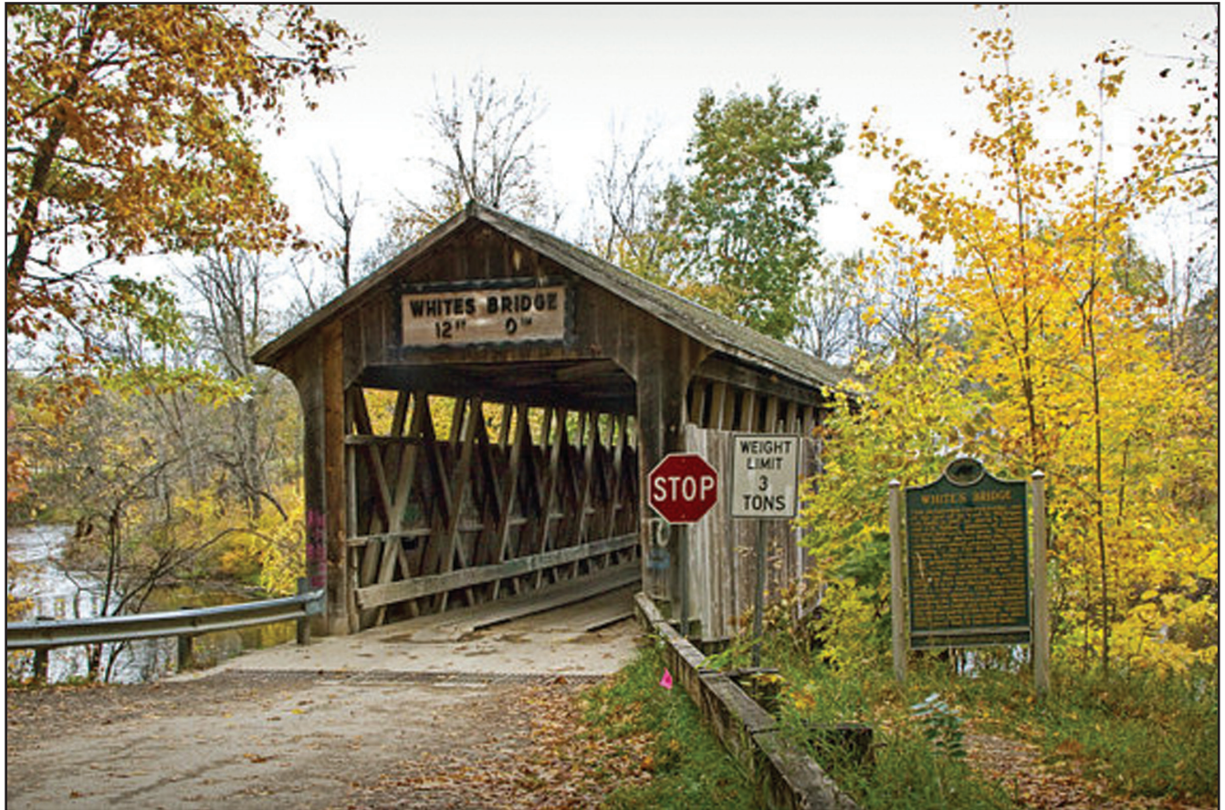
File photo of Whites Bridge before it was burned down by an arsonist on July 7, 2013.
