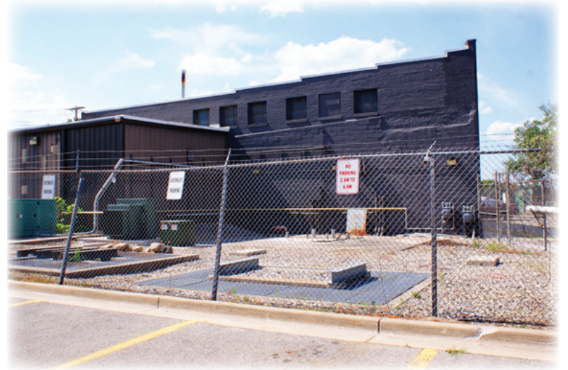
This area behind Lowell Light & Power will soon be the home of a natural gas regulating station.
