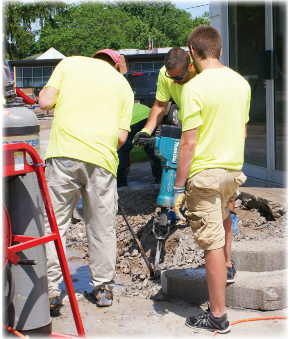
Workers demolishing the church's front steps.
