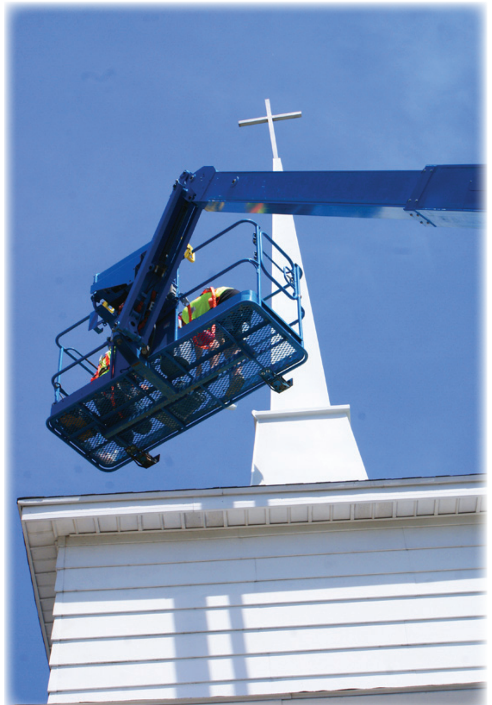
Workers started painting at the steeple and worked their way down.
