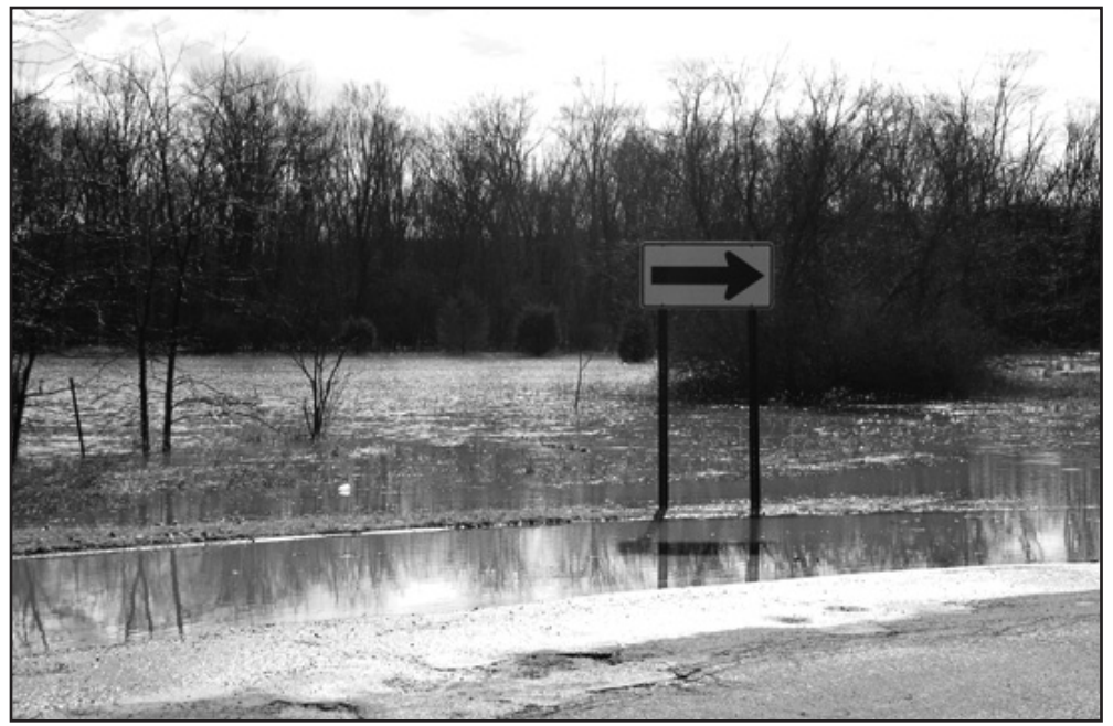
Some streets were impassable, as shown in a photo from the flooding last week.
