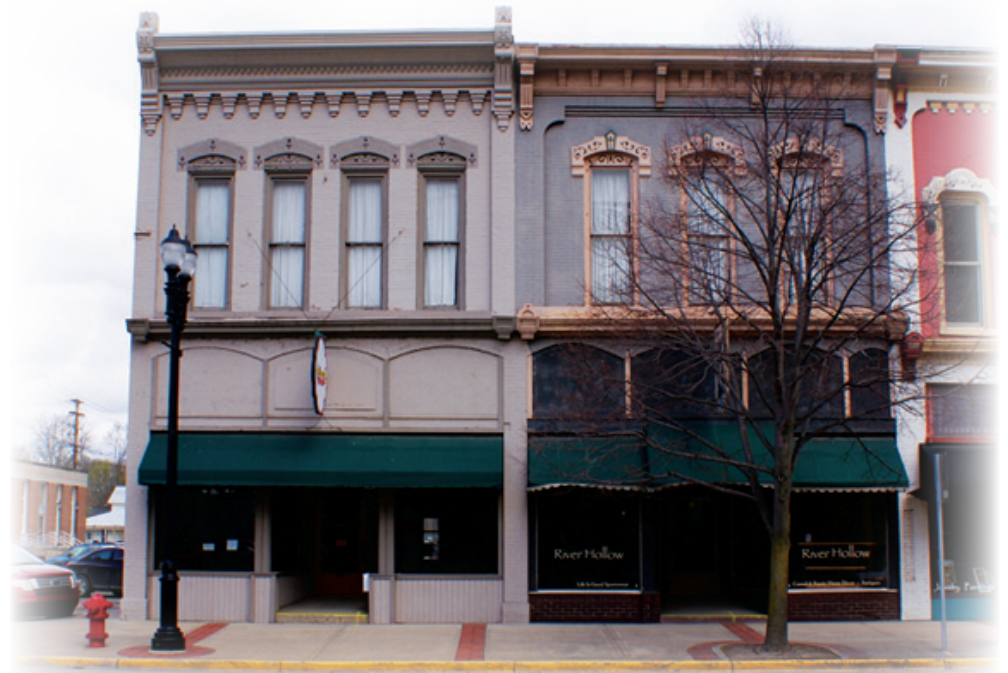
The building has been transformed since this picture taken when LowellArts bought it back in 2015.
