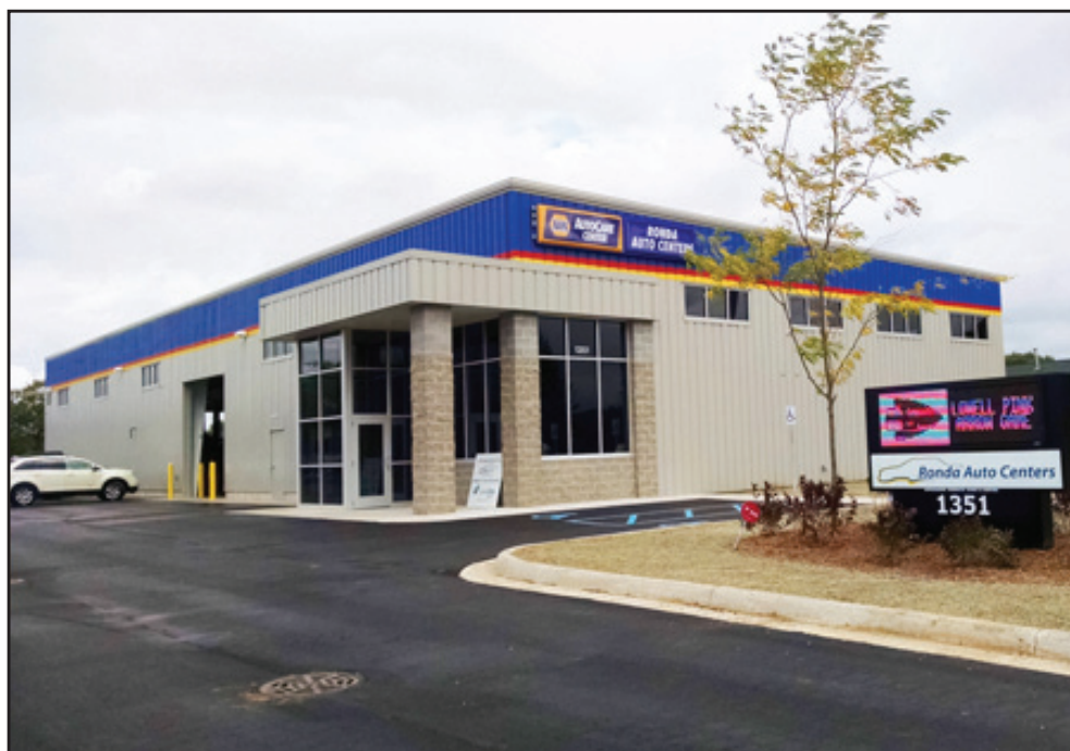
The brand new Ronda Auto Center building at 1351 Bowes Rd. opened its doors last week.
