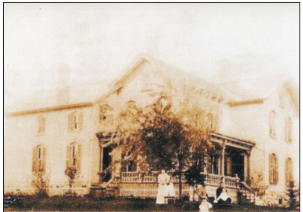
The original farm house that burned down.
