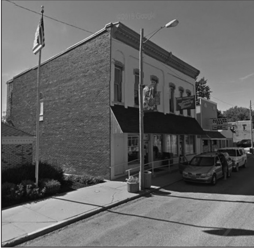
Until three weeks prior, this brick building in Clarksville had housed the community library on one half and a restaurant being refurbished in the other half was set to open in April. (Google Maps image)
