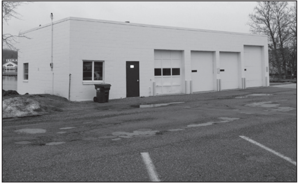
This building at 115 Riverside Dr. was described as "obvious blight" by city manager Burns.
