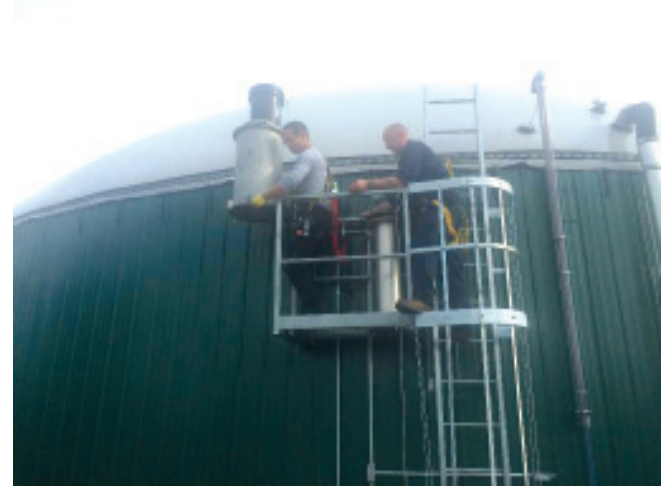
Technicians shown working on biodigester tank. Ledger photo - August 2016
