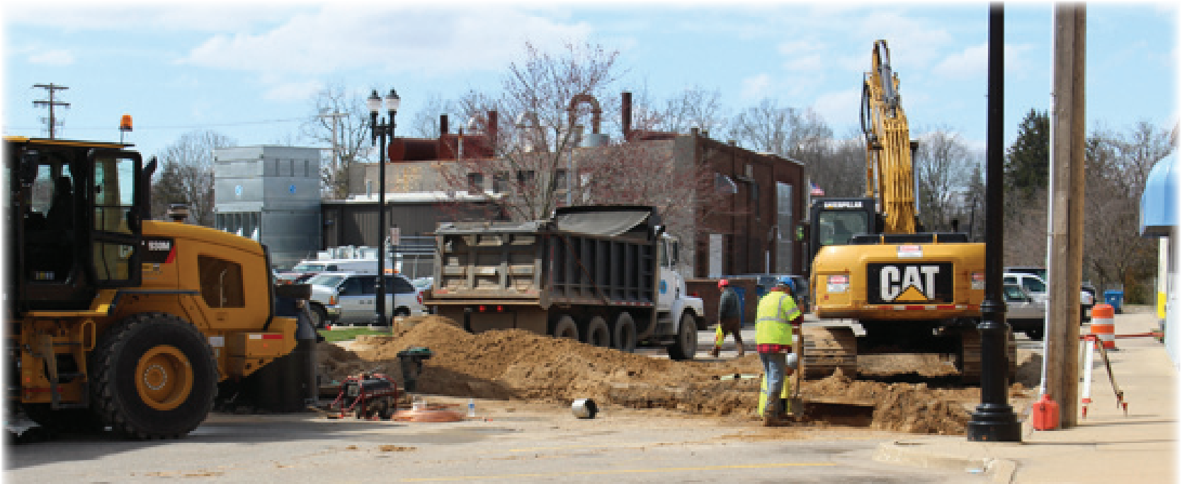
Road crews worked on Riverside Drive in order to replace a sewer line located directly in front of the Backwater Cafe. Work on the one-way road was scheduled to finish yesterday but additional work is scheduled on other local streets. Both Monroe and Avery streets will be under construction throughout the remainder of April. Workers will continue sewer upgrades, resurfacing and improving sidewalks. This is scheduled to be completed prior to the MDOT M-21 resurfacing project.
