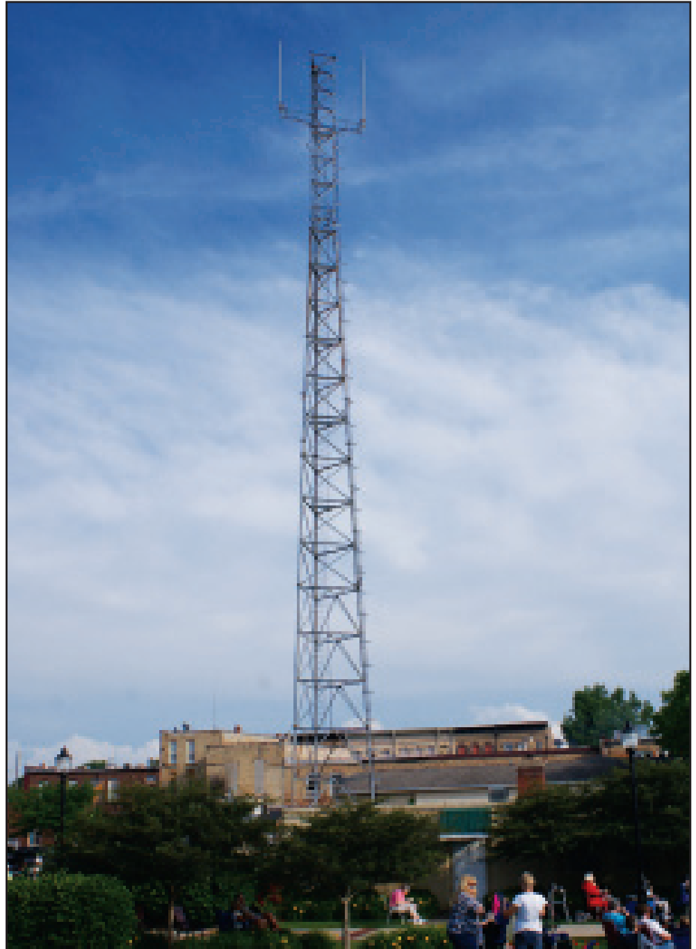
This outdated cell tower in downtown Lowell will be torn down soon.
