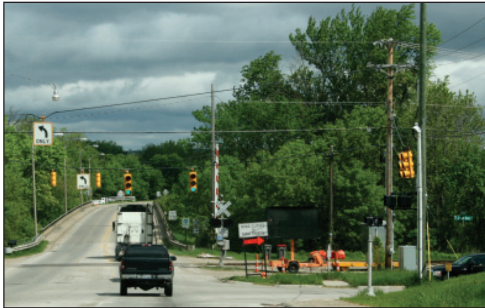
The bridge on Hudson will be closed until July 2.
