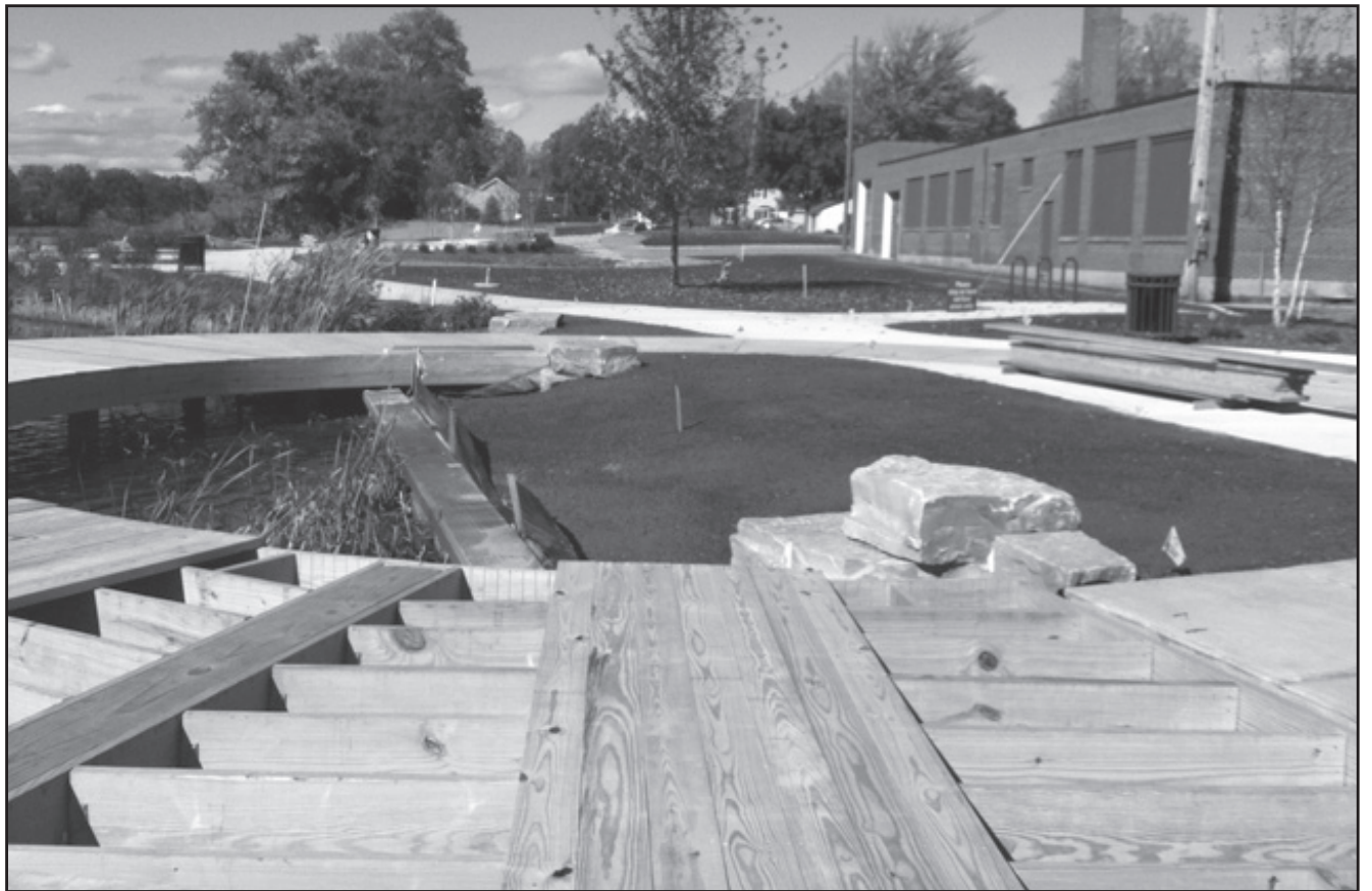
The Riverwalk extension is taking shape.
