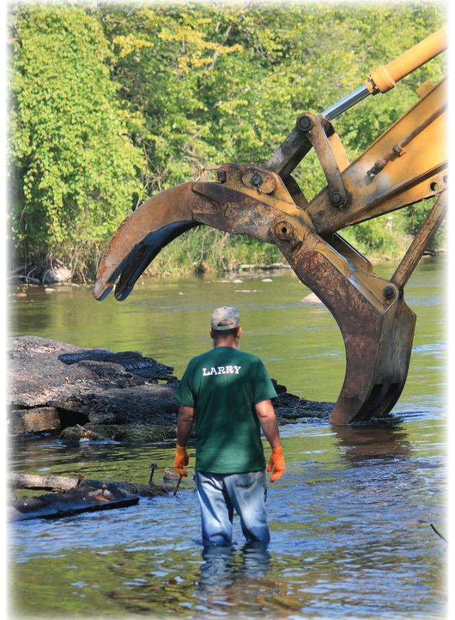
Eco Demolition out of Holland to helped with the clean-up effort.
