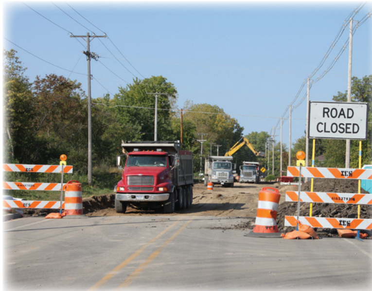
Bowes Road under construction.
