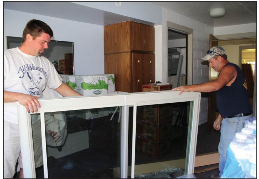
All Weather Seal installs windows at FROM ahead of schedule.
