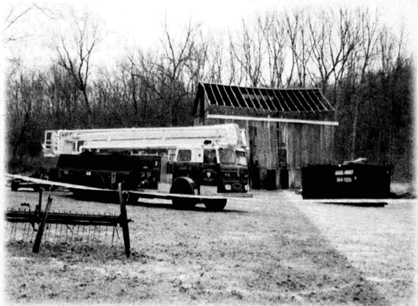
The Tower Farm and barn undergo restoration.
