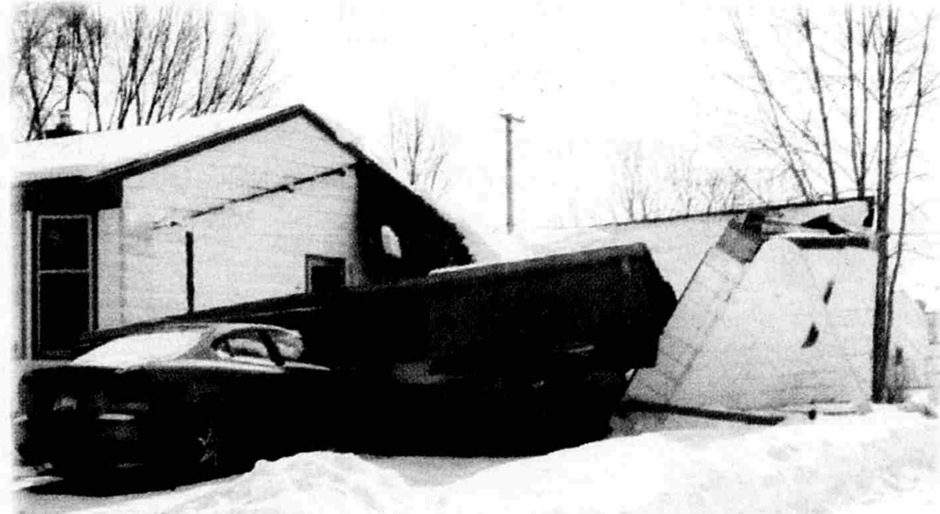
This roof over a garage at a rental home on Valley Vista Drive collapsed due to heavy snow.
