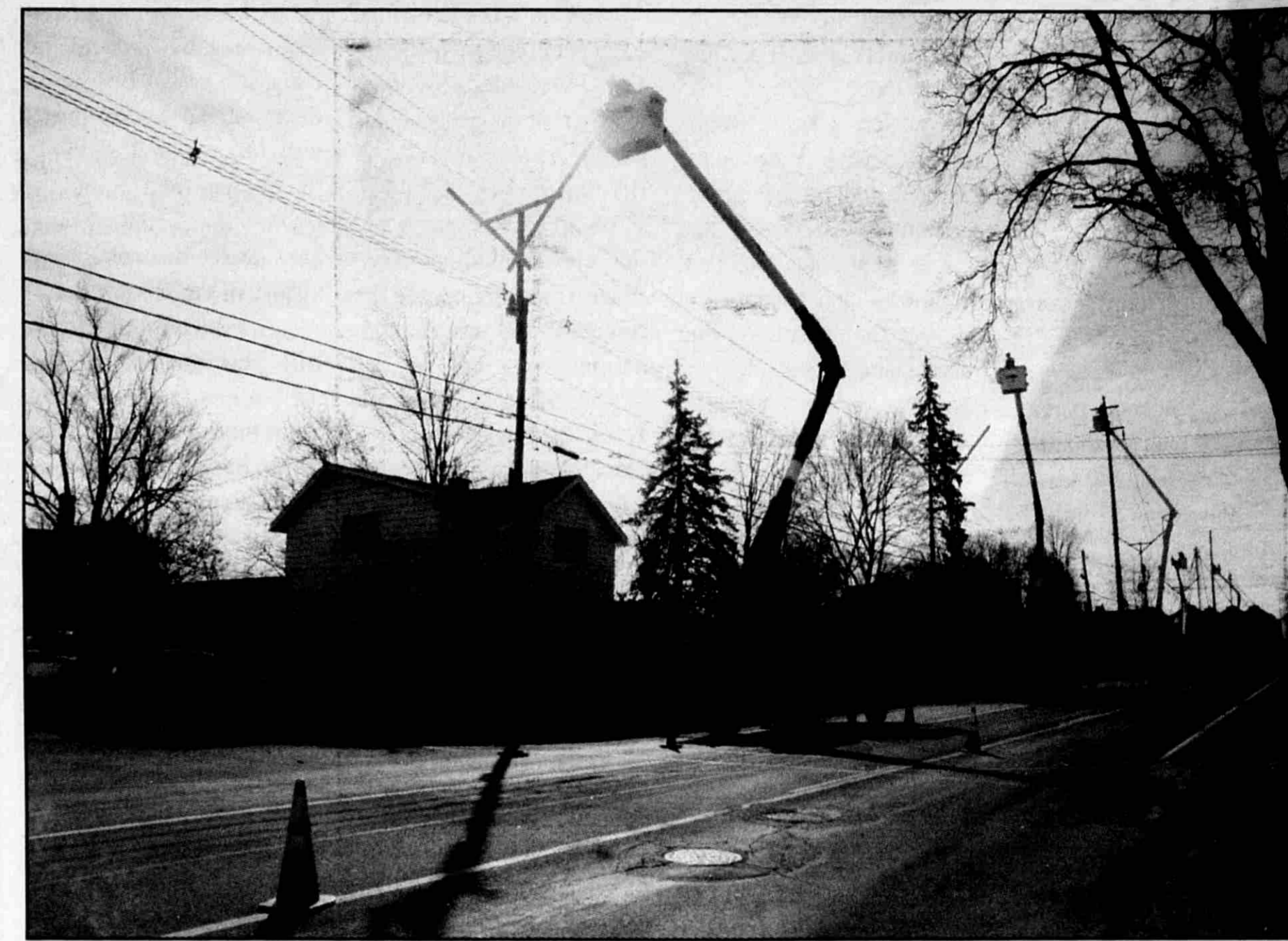
Lowell Light and Power will be putting new poles.
