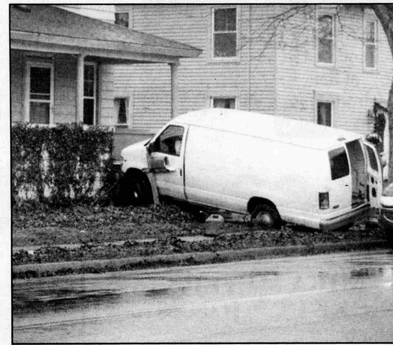
Damage was caused to this home’s porch and railing in a Thursday afternoon accident on Hudson.
