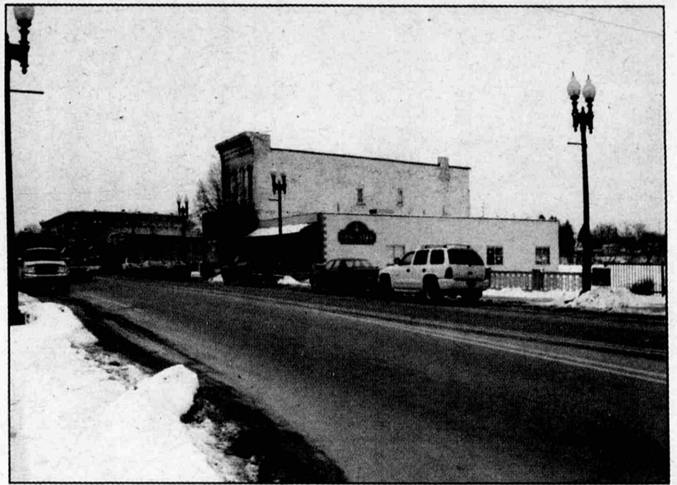
The downtown bridge work to start in mid March, but no detour yet.
